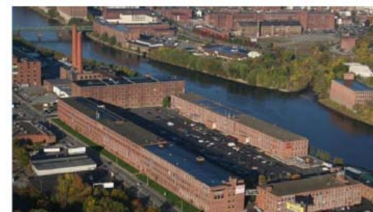
Solectria Renewables, LLC(外観)
