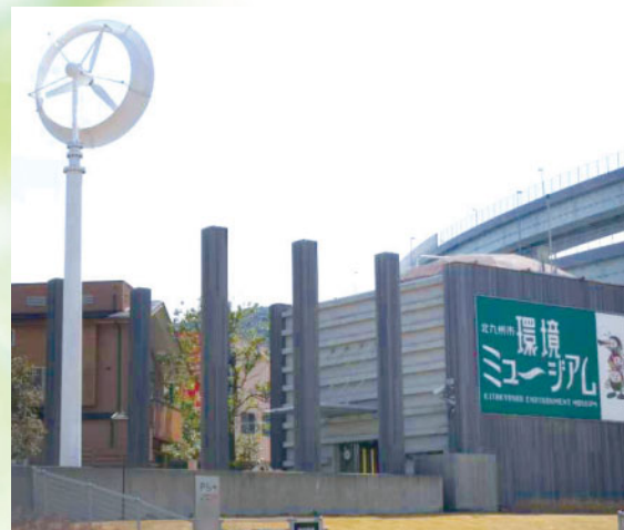
Wind-lens turbine*1 installed at the front entrance (visitors' entrance)
