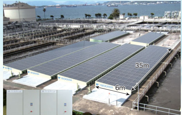
Yaskawa's first high-capacity power conditioner*3 (100 kW × 2 sets)
